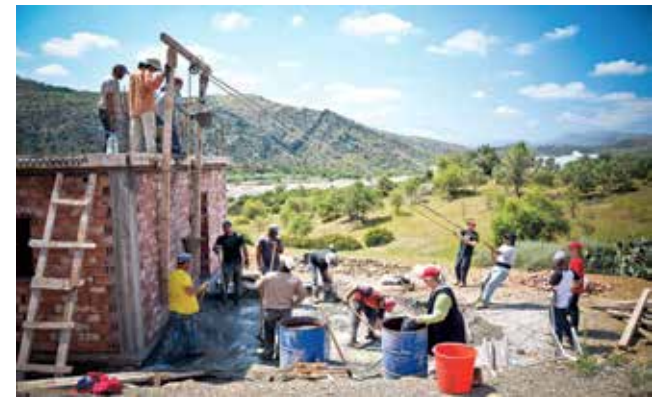
Roofing day. Joseph Easley
