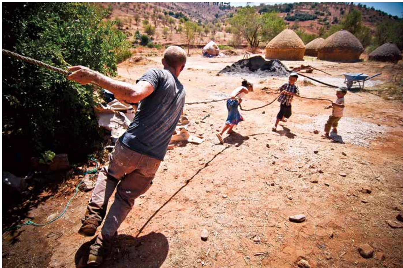
Hauling a bucket of cement up to a roof. Joseph Easley
